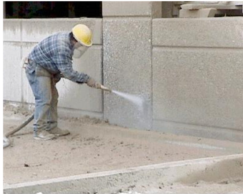
Figure 2. Worker performing abrasive blasting at ground level.
